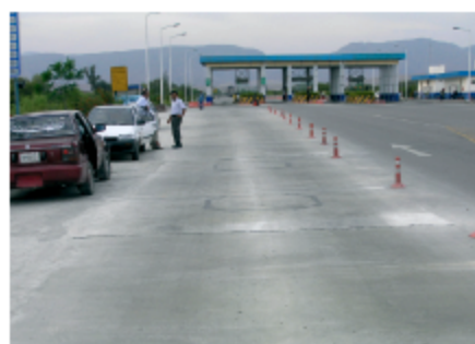
InTeli-WIM provides accurate data of wheel and axle loads as well as gross vehicle weight
